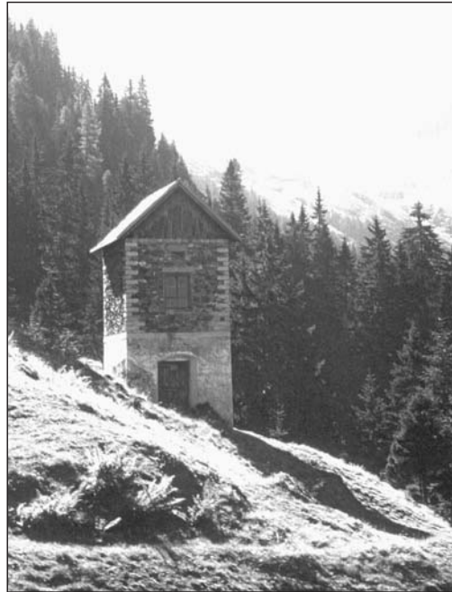
Fig. 5: Explosives magazine of the Kelchalpe mine near Kitzbühel with magazine in the basement and manipulation room in the upper floor (Photo: H. KUNTSCHER 1990).
